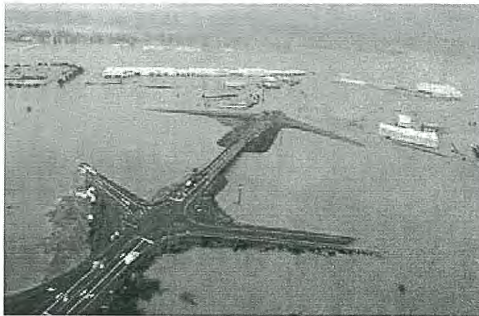
The December 2007 floods completely submerged Interstate 5 in Lewis County. Flooding damaged several area water systems. (Photo courtesy of Washington Department of Transportation.)
