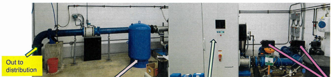
The pressure tank is to dampen surges of pressure from pumps
